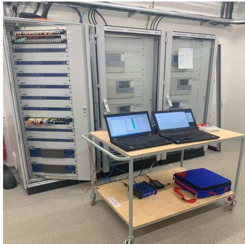
Site Acceptance Test with Omicron Station Scout
